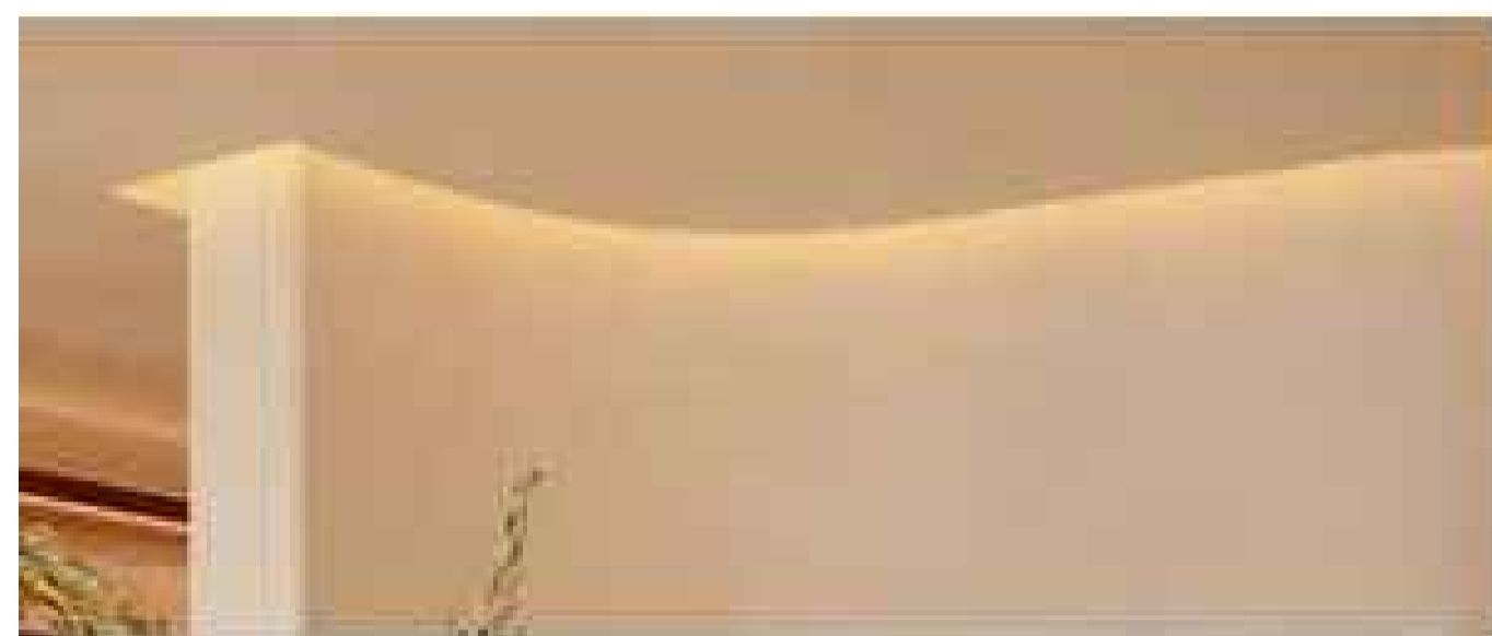
3 Drop Ceiling With Perimeter Inverted Cove Lighting Concept
