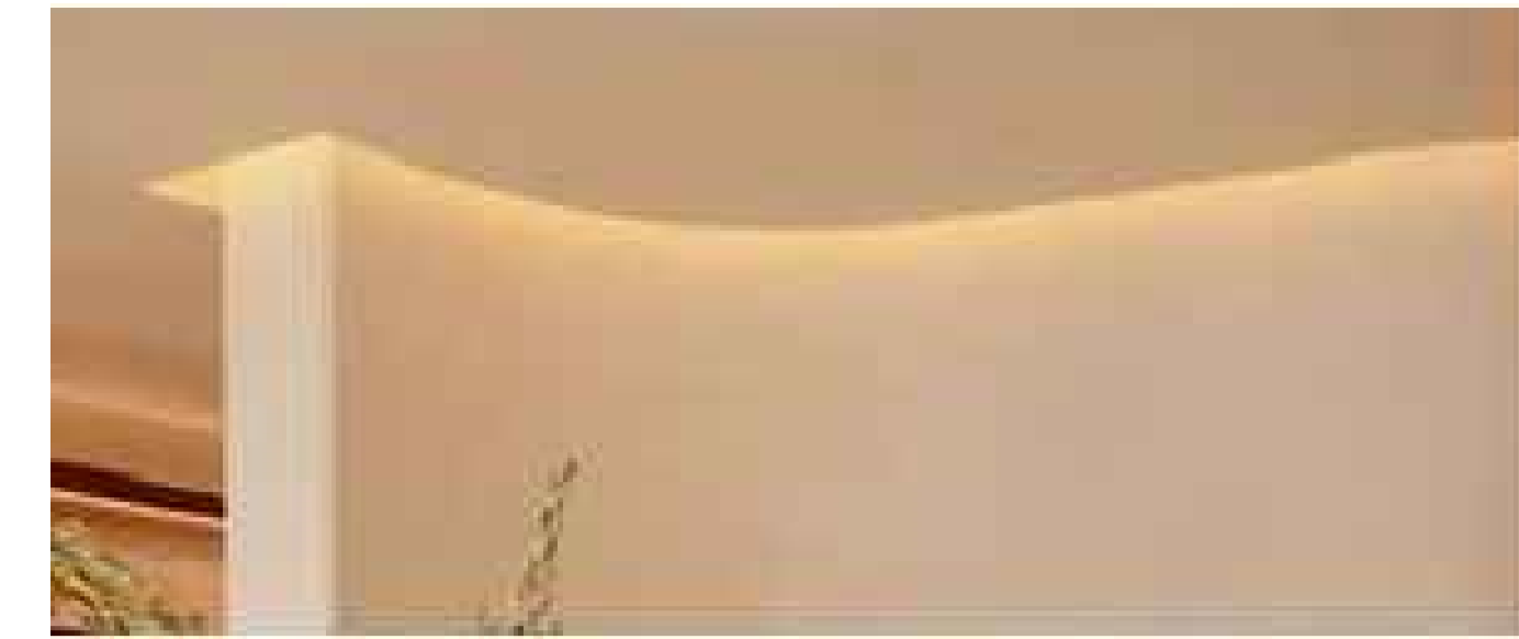
6 Drop Ceiling With Perimeter Inverted Cove Lighting Concept
